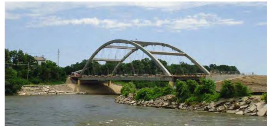
Completed VE Design
